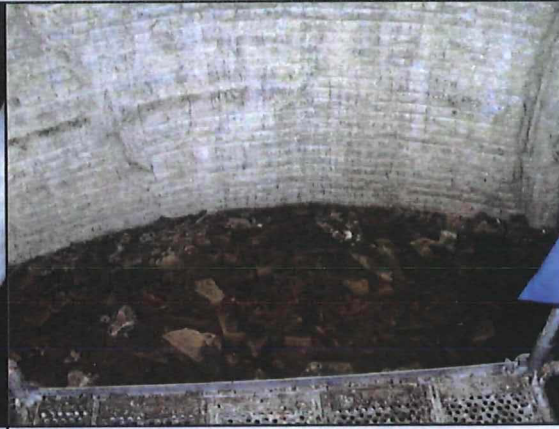
Photo 56: Diffuser Laugenzutritt MP_950-1 (950-m Sohle)
