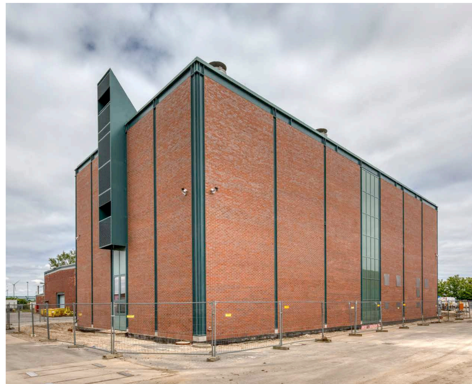
View of the north hoist building, Konrad 1 mine
