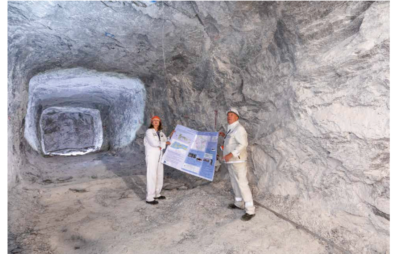
Morsleben repository: Demonstration structure for the permanent sealing of galleries
