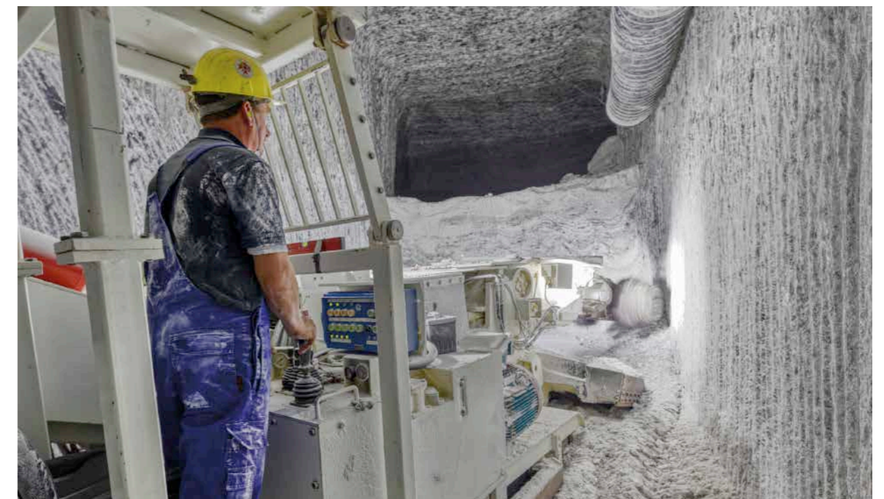
Matthias Bösche creating the backfill site for testing the mixing facility
