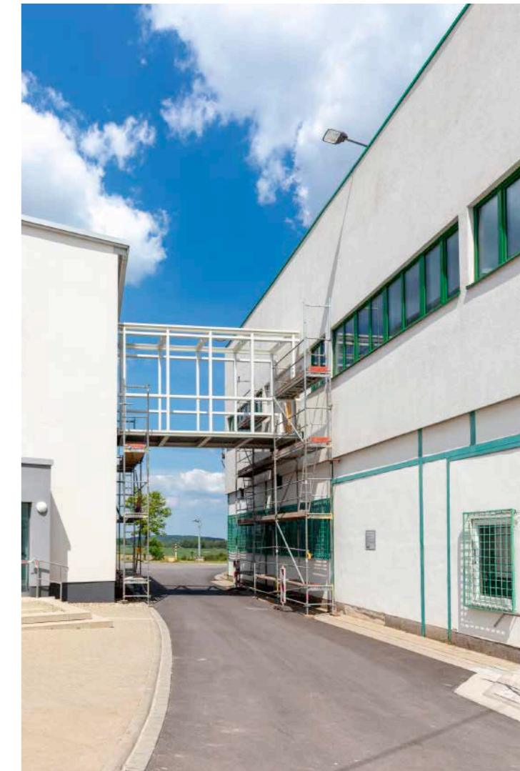
Morsleben repository, supporting structure for the new man-haulage bridge
